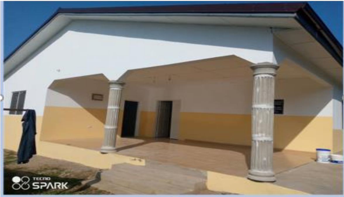
CONSTRUCTION OF 1 NO.8UNITS HOSPITAL WARD WITH OFFICE AT ANUM
